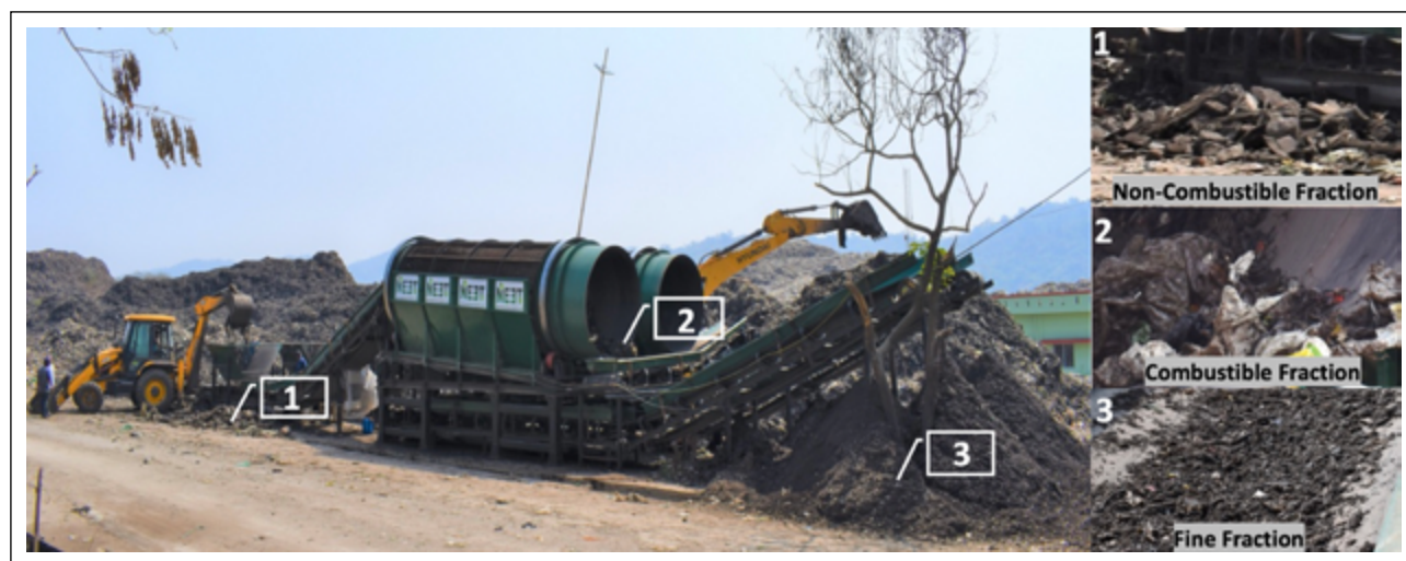
Figure 2. Onsite screening and segregation of the excavated waste.
