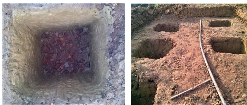
Fig 5. Preparation of composting pit
